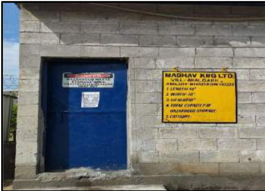
Photograph showing Hazardous waste storage area
