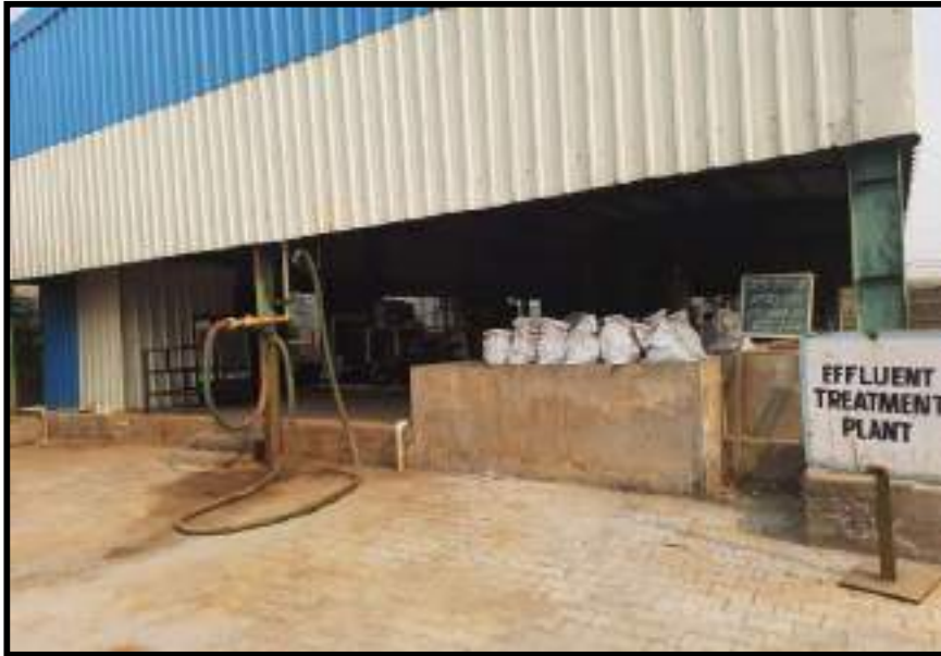
Photographs showing Effluent Treatment Plant
