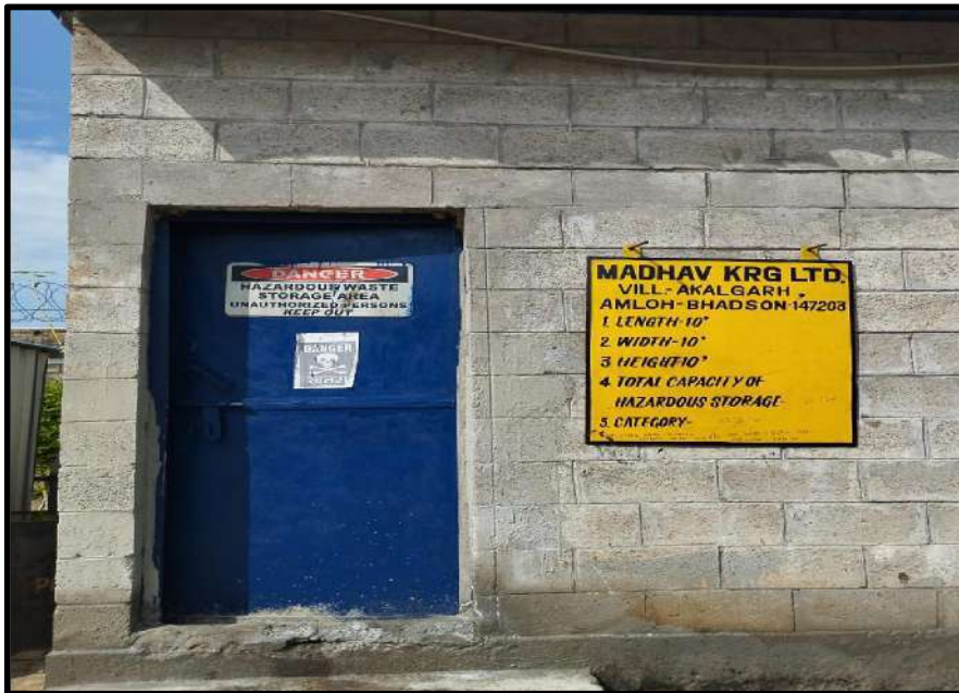
Photograph showing Hazardous waste storage area
