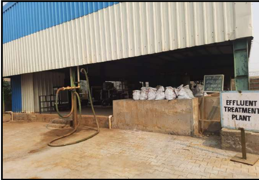
Photographs showing Effluent Treatment Plant
