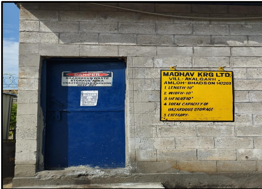
Photograph showing Hazardous waste storage area
