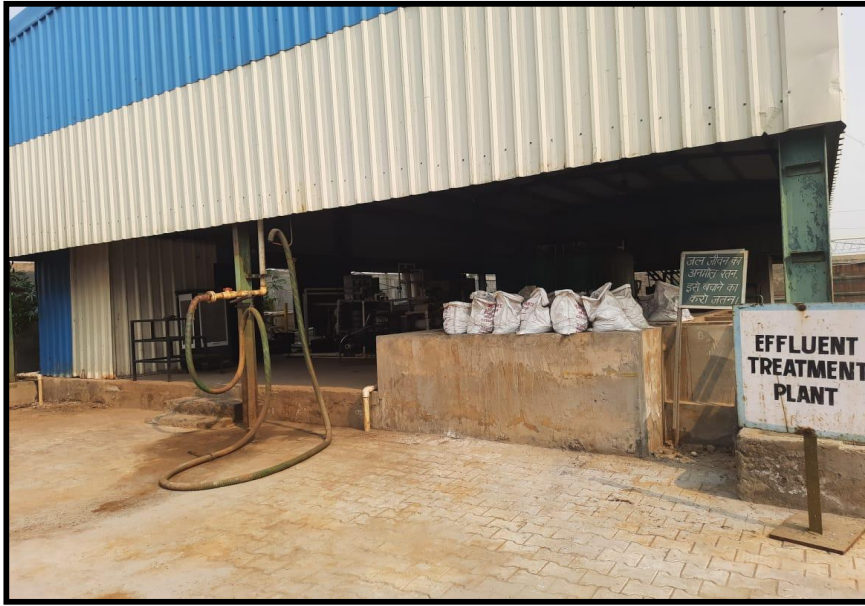
Photographs showing Effluent Treatment Plant
