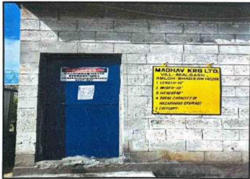
Photograph showing Hazardous waste storage area
