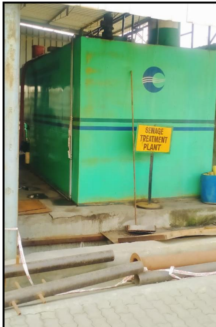
Photographs showing Sewage Treatment Plant
