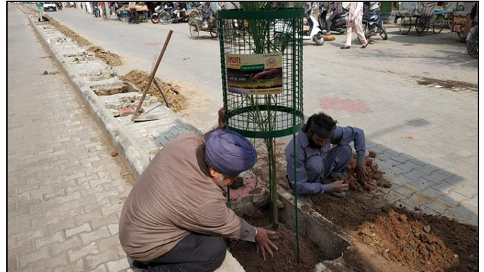
Tree Guard Installation
